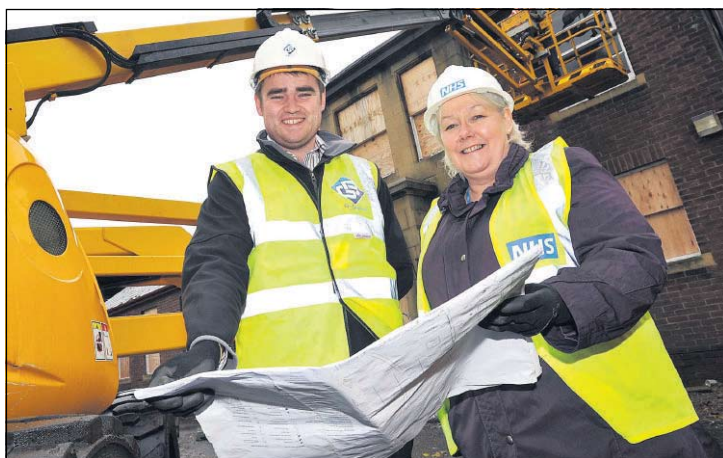
Fran McGrath, site manager for GB Building Solutions Ltd, and Jean Sharp, project officer for Northumbria Healthcare NHS Foundation Trust, pictured before the demolition of Haltwhistle War Memorial Hospital.
